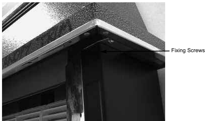
Fig. 7 Removing the Upper Outer Case Fixing Screws
