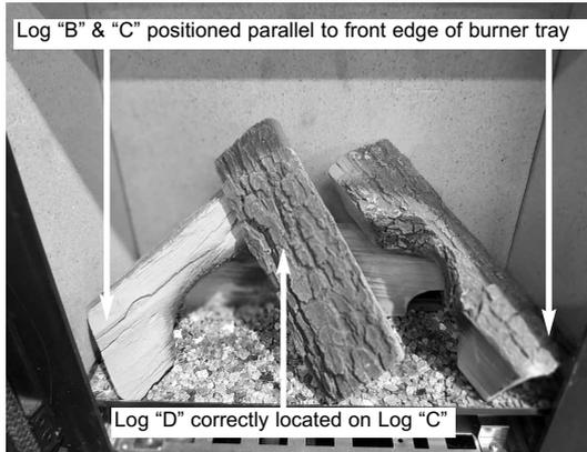
**IMPORTANT NOTE :** ENSURE THAT THE LOGS "B" & "C" ARE POSITIONED SO THE FRONT CORNERS OF THESE LOGS ARE PARALLEL WITH THE EDGE OF THE BURNER TRAY AS SHOWN ABOVE IN FIGURE 20.
