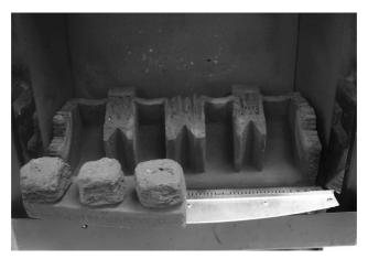
c) Place the right hand front coal rail moulding onto the front ceramic rail support as shown below in figure 3.
