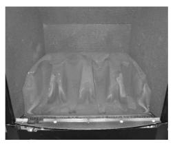
b) Position the two halves of the front ceramic (L/H & R/H) on the locating channel in the front ceramic, ensuring it is located onto the lip on the burner front ceramic support. (See figure 15 below)
